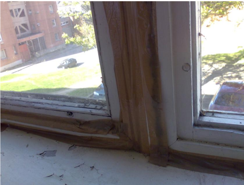
Picture 4. Temporary window insulation made with tape.
